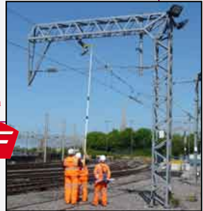
NETWORK RAIL - Angleterre
